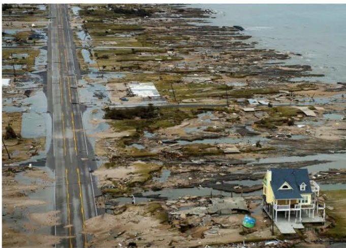
BOLIVAR PENINSULA IN TEXAS AFTER HURRICANE IKE (2008)
