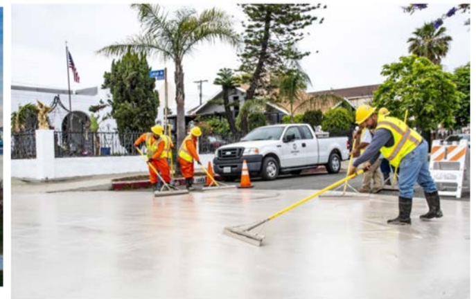
Workers apply CoolSeal to a street in Pacoima in June. Los Angeles Bureau of Street Services
