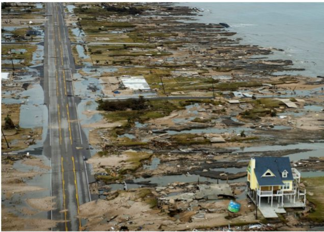
BOLIVAR PENINSULA IN TEXAS AFTER HURRICANE IKE (2008)
