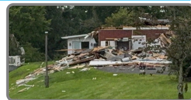
Damage from an EF-2 tornado in West Virginia on July 21. Credit: NWS RLX
